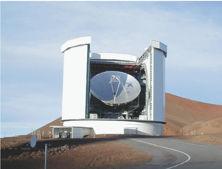
Fig. 1.23. The JCMT has a 15-m dish. It is protected by the largest single piece of Gore-Tex, which has a transmissivity of 97% at submillimeter wavelengths
